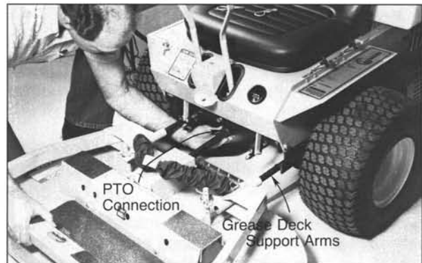
PHOTO 3-6 Mower Deck Installation (PTO Shaft Connection)
